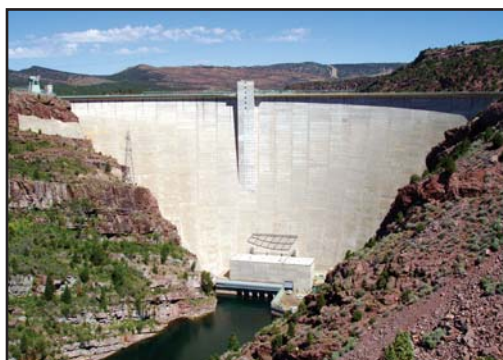
Hydroelectric Turbines, Flaming Gorge Dam
